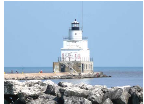
Mantiwoc Breakwater WI Loc: Mantiwoc Const: 1918 Tower Ht: 40' Status: Active
