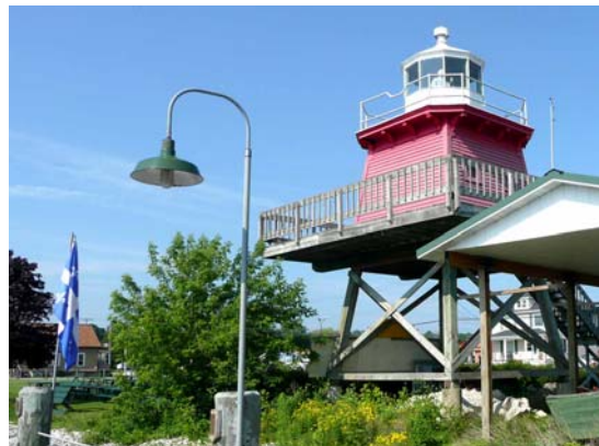
Two Rivers WI Loc: Two Rivers Const: 1928 Tower Ht: Status: Inactive
